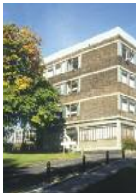
Crawford Theatre, University of Strathclyde, Scotland The roof was prohibited from being subjected to additional loading. The use of the Kingspan KoolDuct® System reduced the overall service loading, and the consequent design strength (and hence cost) of the steel support system.
